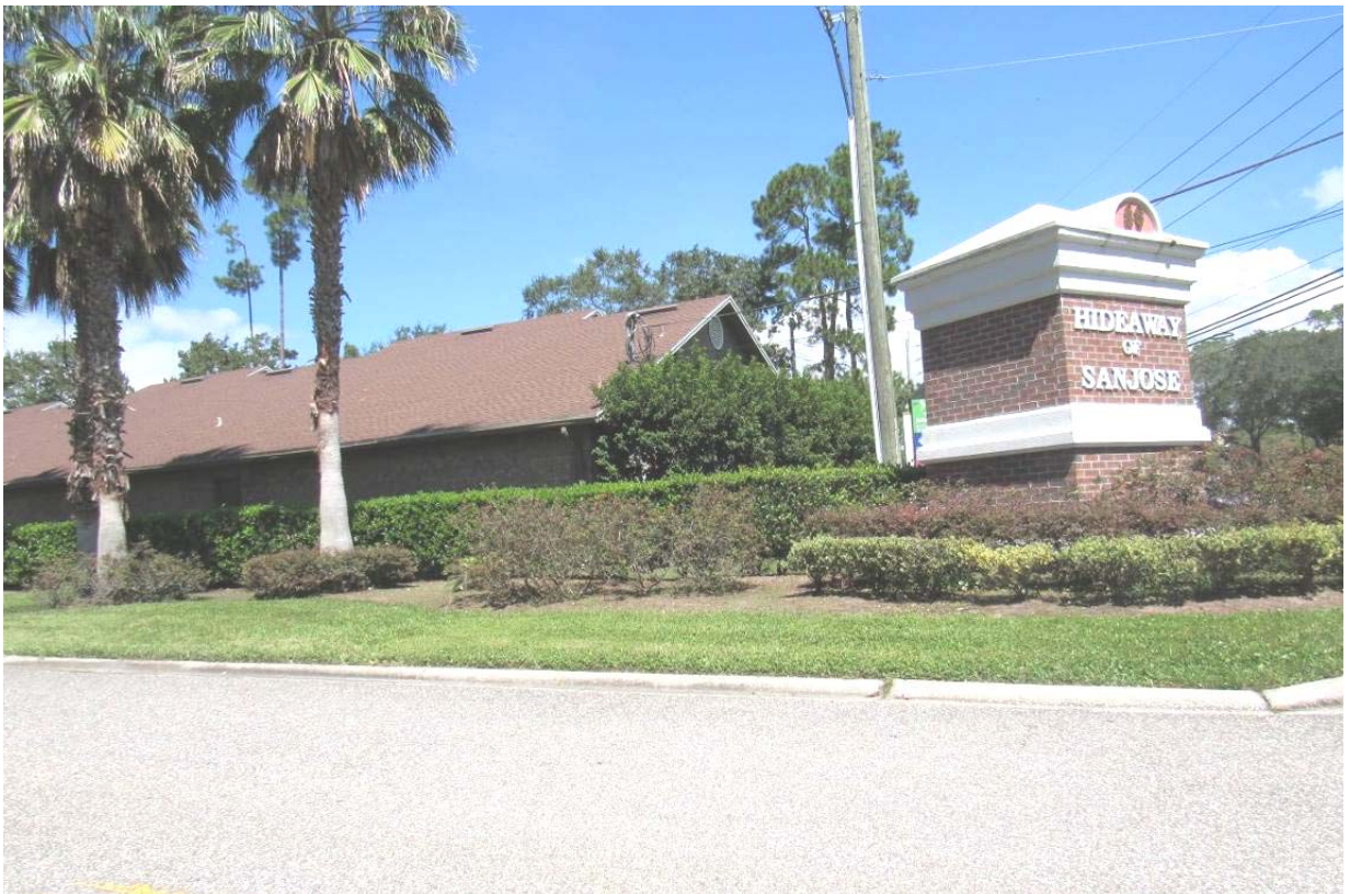
View of adjacent office building
